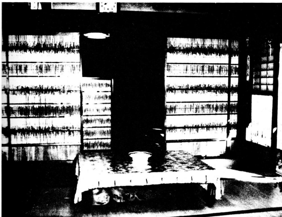
Fig. 1. Sliding doors and an interior shading blind made of reed in a Japanese style house.
